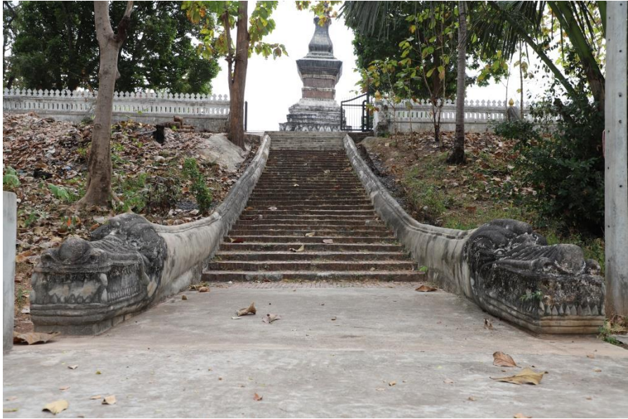
The southern staircase. The photograph was taken on 23 January 2024 by Khamvone Boulyaphonh.
